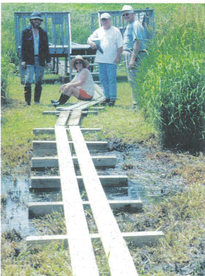
Left to right: David Homan and Ethyle McClelland (Stewards), Bob Bryan, and Bill Smith build a much-needed boardwalk thru a swampy section of the Ropchan Wildlife Refuge. Sean Carroll, Carl Deimling and Bob Bryan transported the lumber to the site and the work was completed on one very muddy morning. Thank you!
