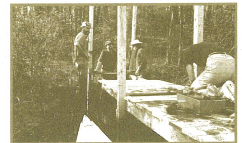
Above: Peter Martin, Douglas Eberhardt & Ron Hendel work on the dock at Wing Haven.
